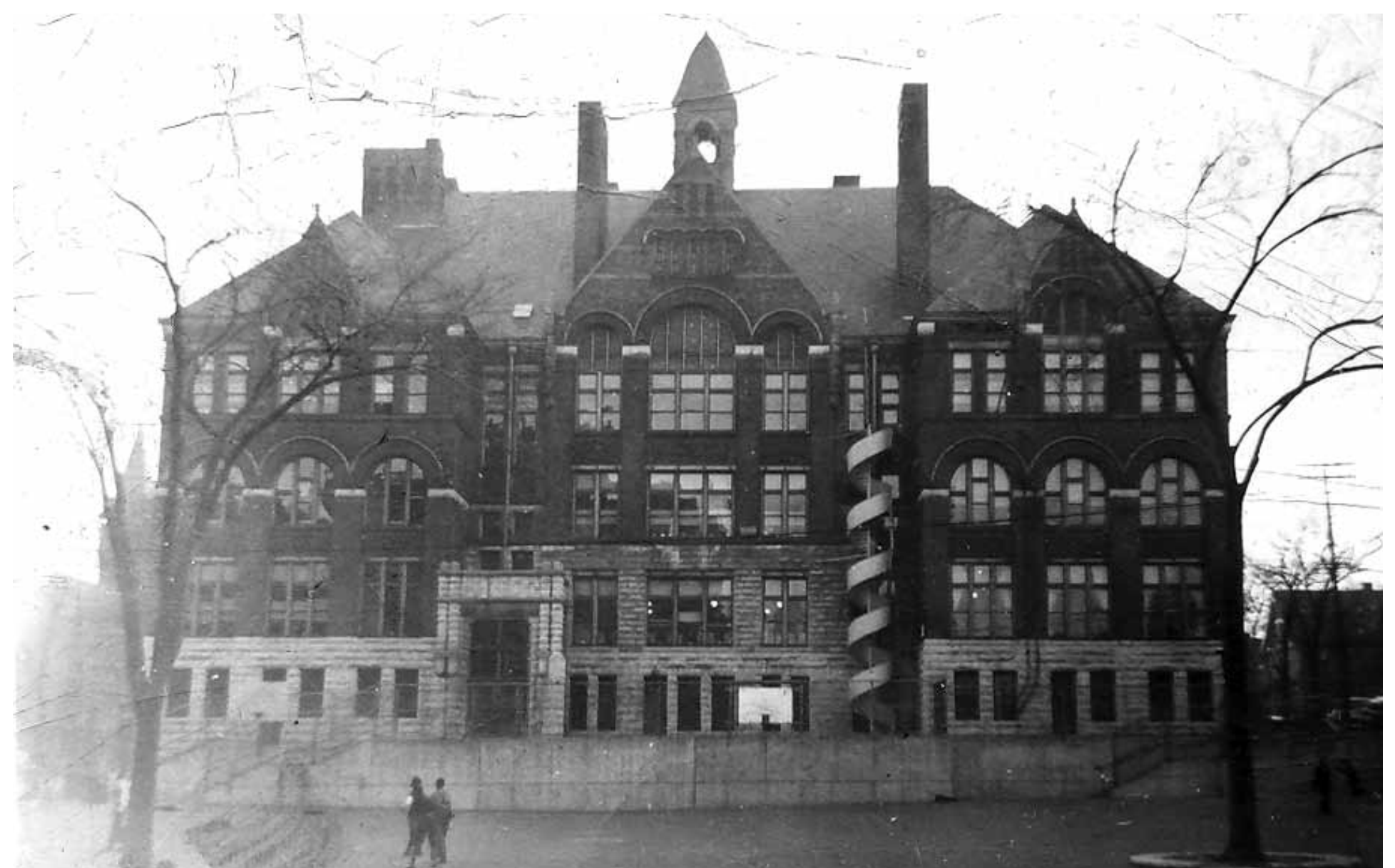
The Ninth Street School was torn down in the 1960s for construction of Highway 43. Photograph courtesy of Larry Miller.
